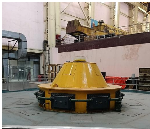
Fig.5 Unit 1 Generator
